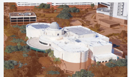
Identify RF Ground-Based Obstructions
